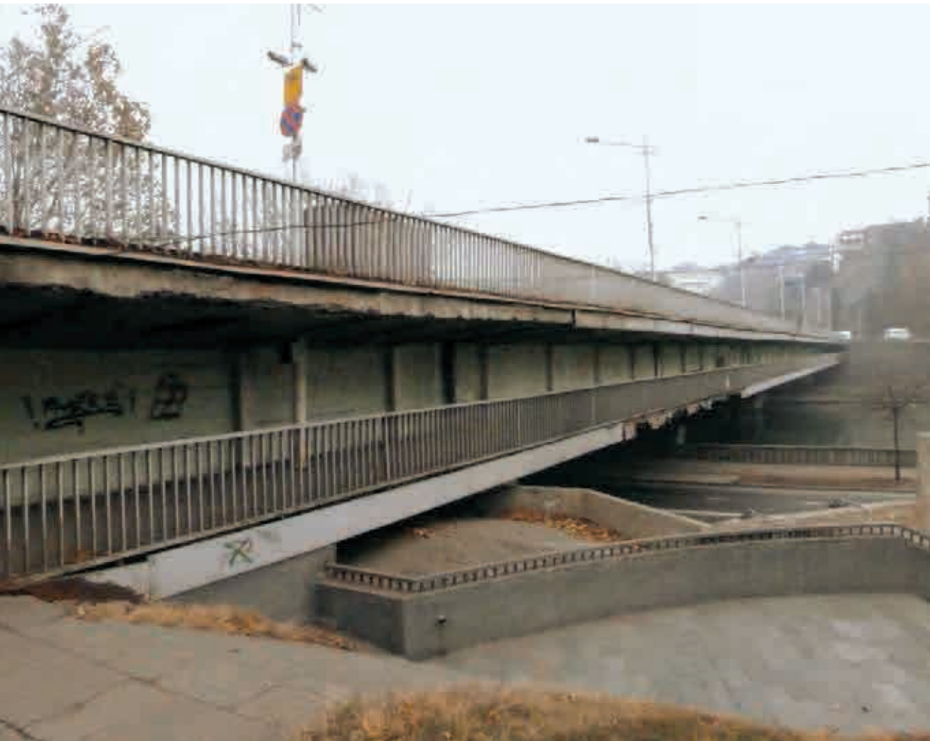
Baratashvili Bridge and underground passage, Tbilisi, 2012. Photo by Nini Palavandishvili
